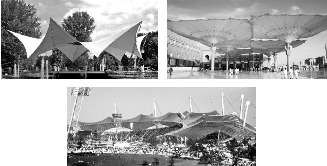
Figure 1. Iconic double-curved freestanding canopies: Tanzbrunnen in Köln (1957, upper-left, SL-Rasch), Olympic Stadium Roof in Munich (1972, lower-center, SBP), Haram Plaza in Medina (2010, upper-right, SL-Rasch).
